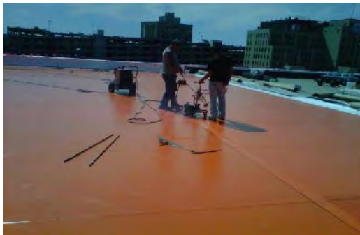
Application of Roof Membrane
